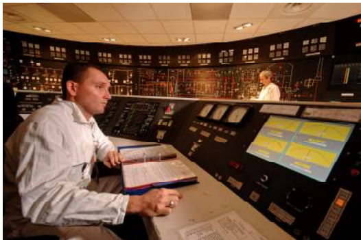
The control room of Orphée reactor
