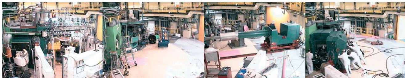
Figure 5. 4 steps of the works on beam tube 4. From left to right; 3T2, 4F1 and 4F2 in operation in June 2006, empty space beginning of July, thimble testing mid-July and 4F1-4F2 monochromator protection back in place in September.
